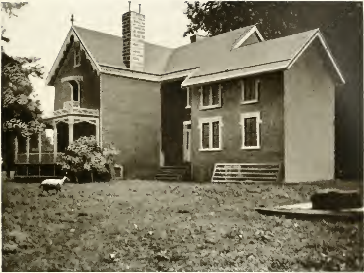
DOWNMAN HOUSE NEAR FREDERICKSBURG, VIRGINIA.
