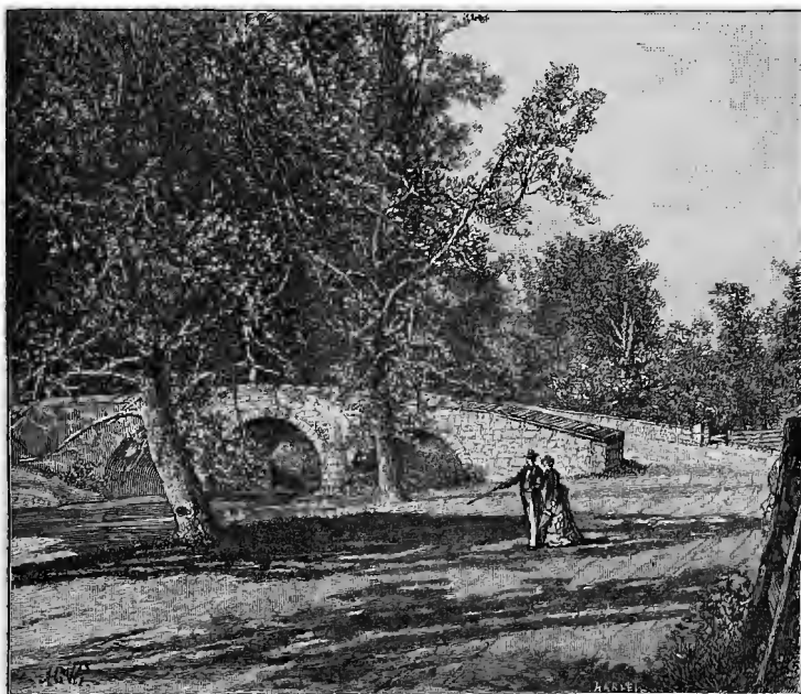
THE BURNSIDE BRIDGE OVER THE ANTIETAM.
