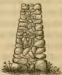
A SECTION OF WALL IMPROPERLY LAID.
